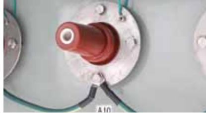
High Voltage Separable Connectors
